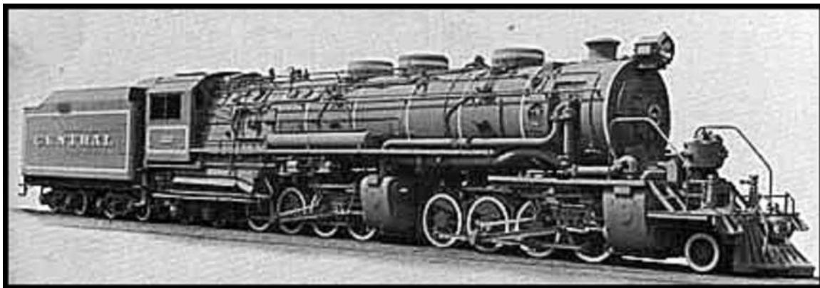
This 1937 Henschel-built 2-8-8-4 had the largest boiler of any narrow gauge engine.
