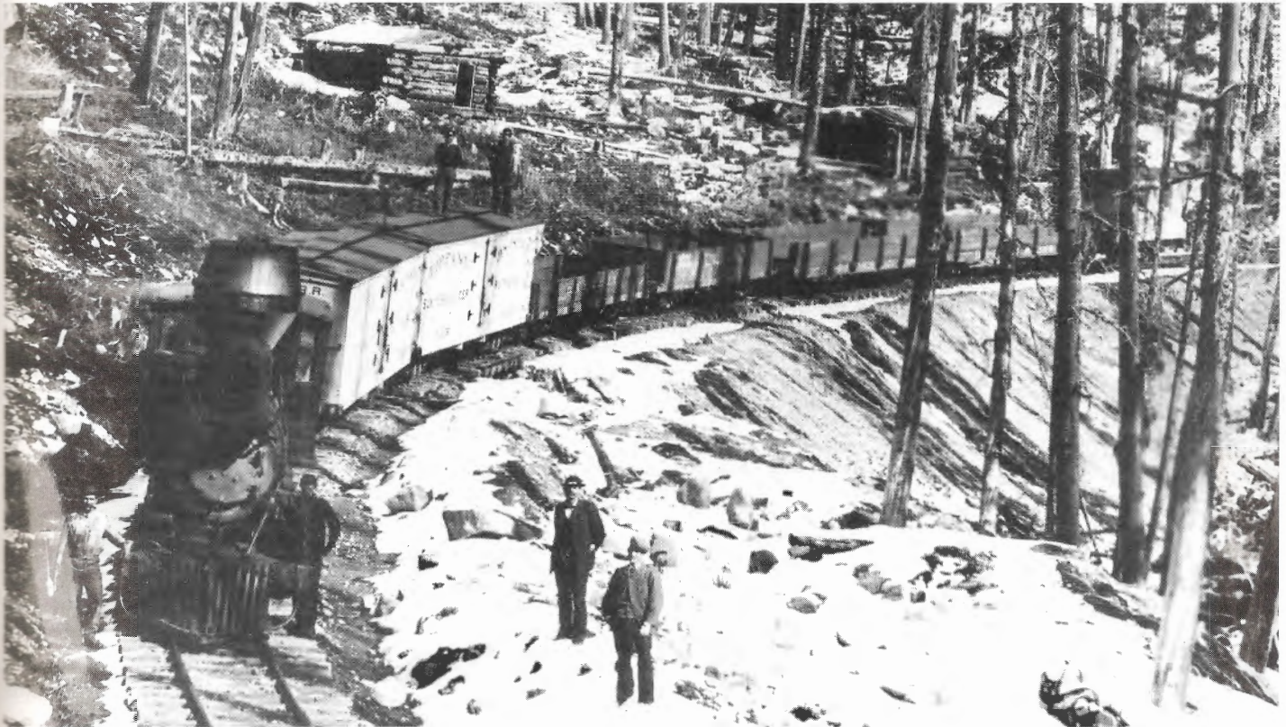
Photo 3. One of two very clear William Henry Jackson photos of Tiffany reefers 1064 and 1057 from about 1888 plainly illustrates the lack of roof hatches, even under powerful magnification. The location is Hairpin Curve at Alpine Pass below Woodstock on the western approach to the Alpine Tunnel.
