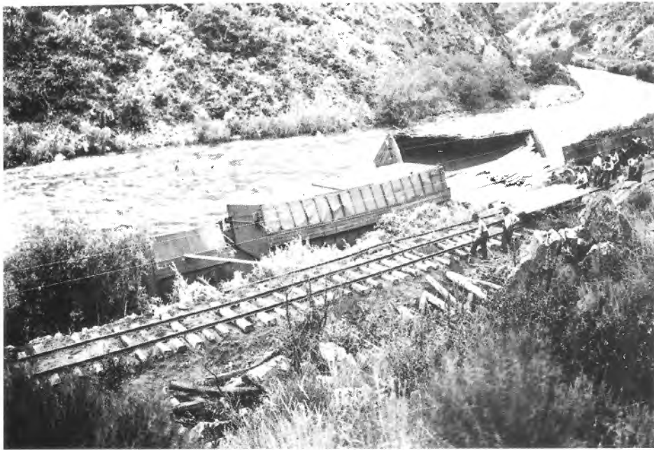
Photo 2. The unidentified caboose in this July, 1912 wreck may be the earliest example of a rebuilt C&S caboose. The end ladder has straight frames and the roof ends have no lateral roofwalks.
